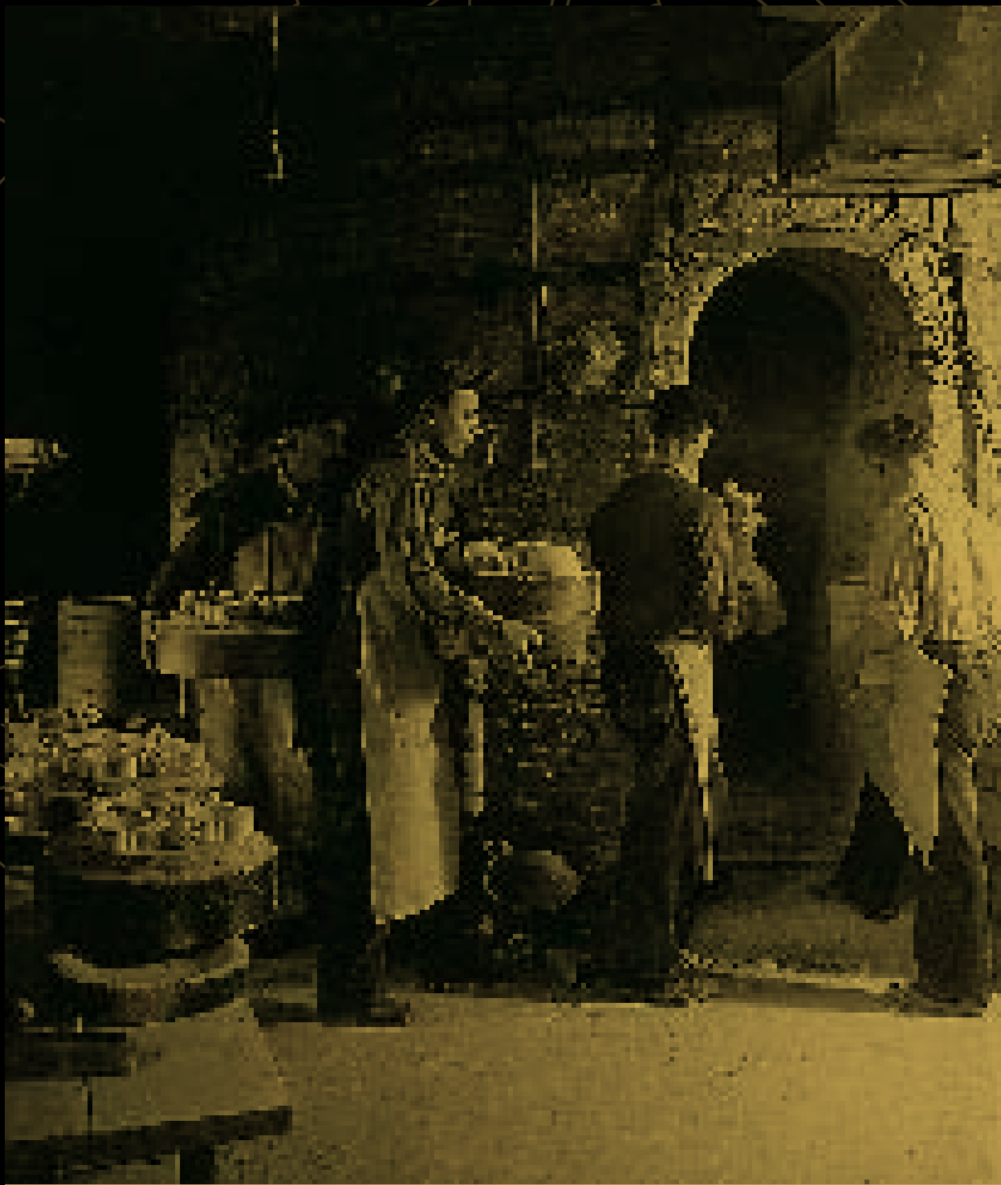
The lining of the muffle before the first firing, porcelain baker Ferenc Trum Photo: Ernő Vadas, 1953-54 (Archive of the Museum of Applied Arts)
